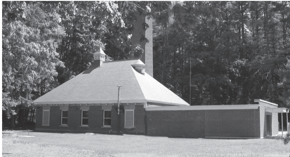
Baddacook Pond Treatment Facility
