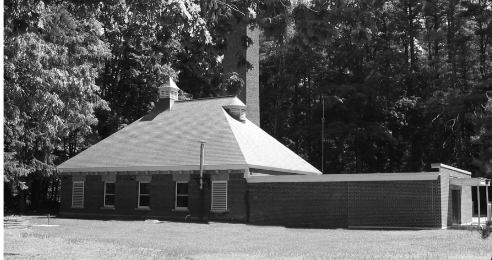
Baddacook Pond Treatment Facility
