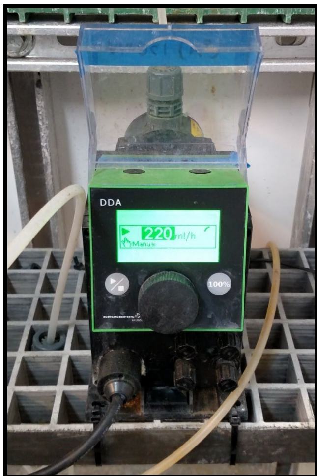
Figure 2.07: Sodium Hypochlorite Feed Pump
