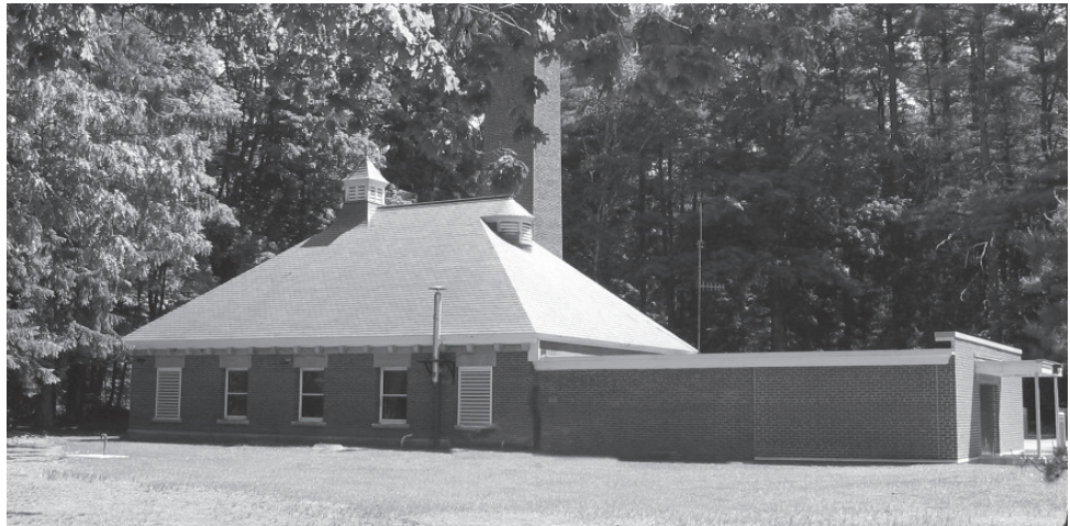
Baddacook Treatment Facility
