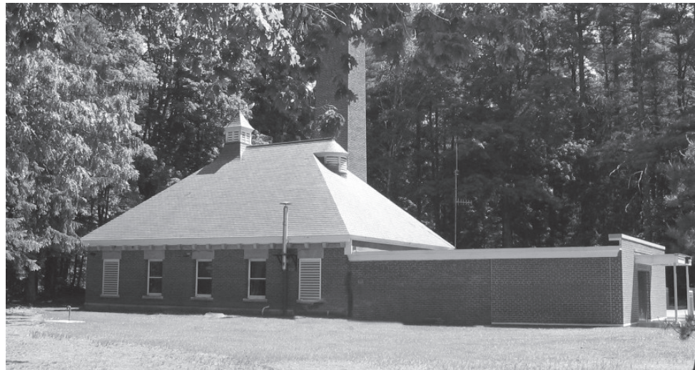
Baddacook Pond Treatment Facility
